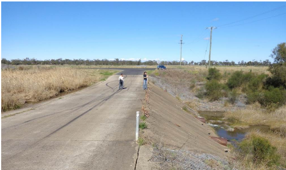
Figure 5. Drop structure at Wallingford Road.
